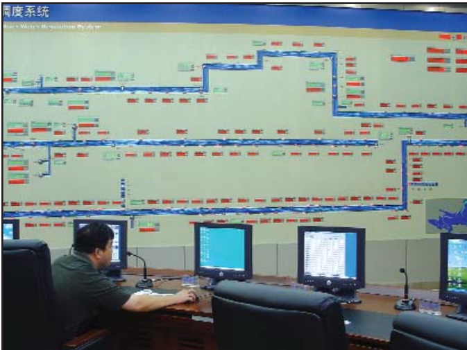
An operator accesses the Yellow River's plant intelligence and supervisory control system through the Industrial Application Server Integrated Development Environment.
